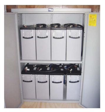
This battery enclosure allows for stacking batteries, reducing the footprint required. This is one clear benefit of sealed batteries, as access to cell caps to add water is unnecessary.
